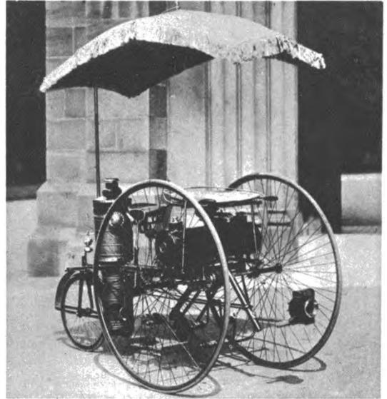
6. In 1886, New Jersey's Lucius Copeland built this handsome steam tricycle. Weighing 185 pounds and with a surrey-type fringed top, the machine seated two in tandem, was equipped with pedals to help the steam engine on hills. Unfortunately, nothing remains of Copeland's famous tricycle but this rare old photograph.
