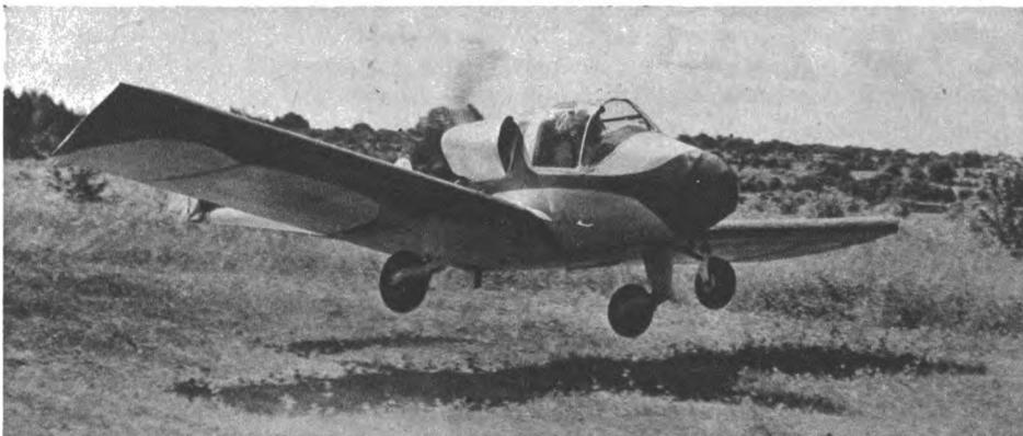
Car, now a plane, goes aloft. It can stay up over three hours, cruises at 90 mph. What a way to get to work!
